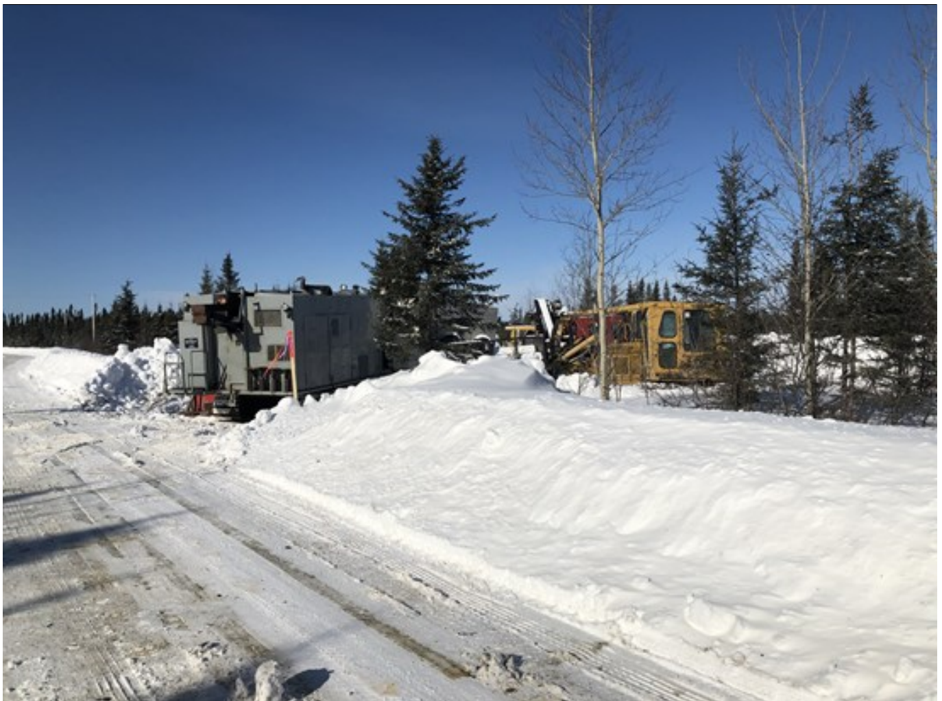
Fig. 2: Drill arriving at site, being mobilized to NW zone.
